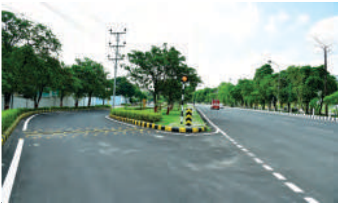
To ensure proper road visibility, rumble sheets were placed across the 6km stretch in Greater Noida, UP
