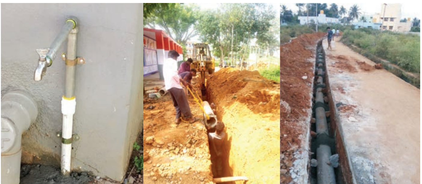
Underground drainage and drinking water lines laid down for 450 households in Mindahalli and Karinyakanahalli villages in Karnataka
