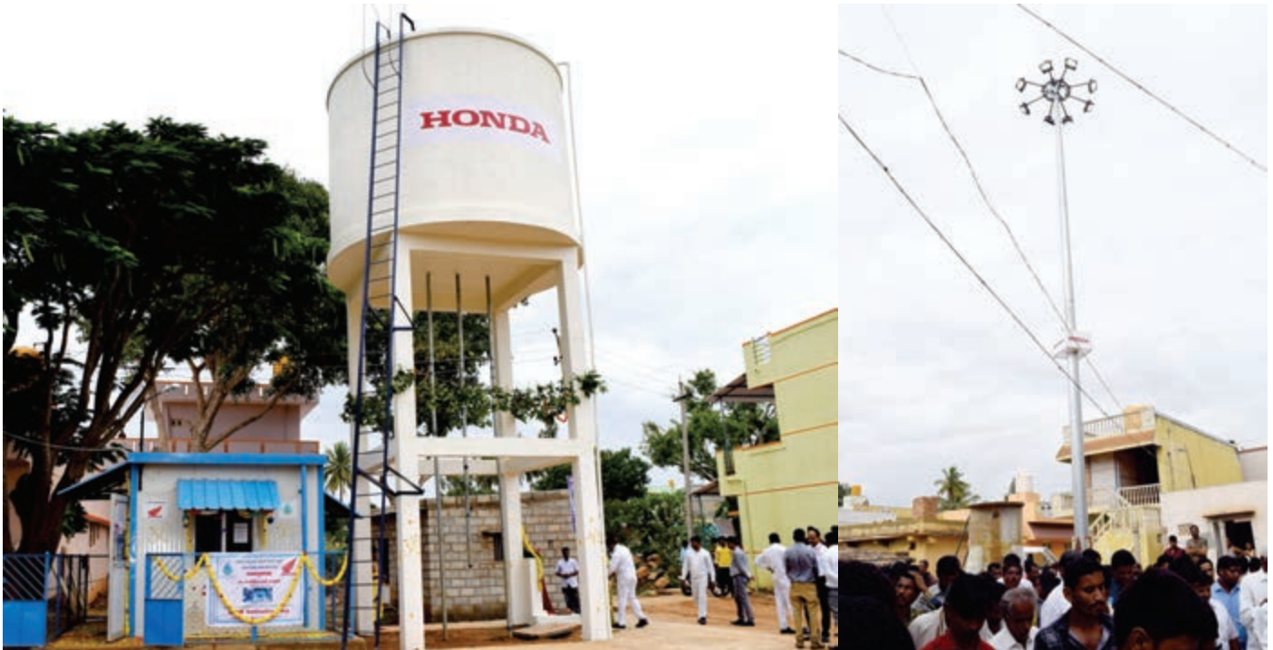
Community water RO plant, Overhead water tank & high mast light at Karinayakahalli & Mindahalli, Karnataka
