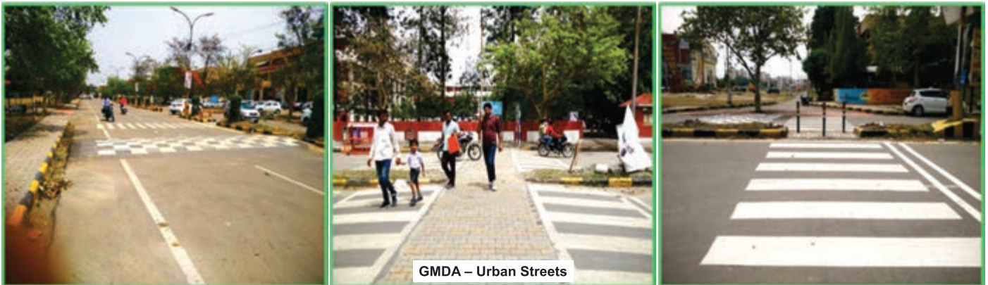
Road Safety signage and construction as part of HVZ
